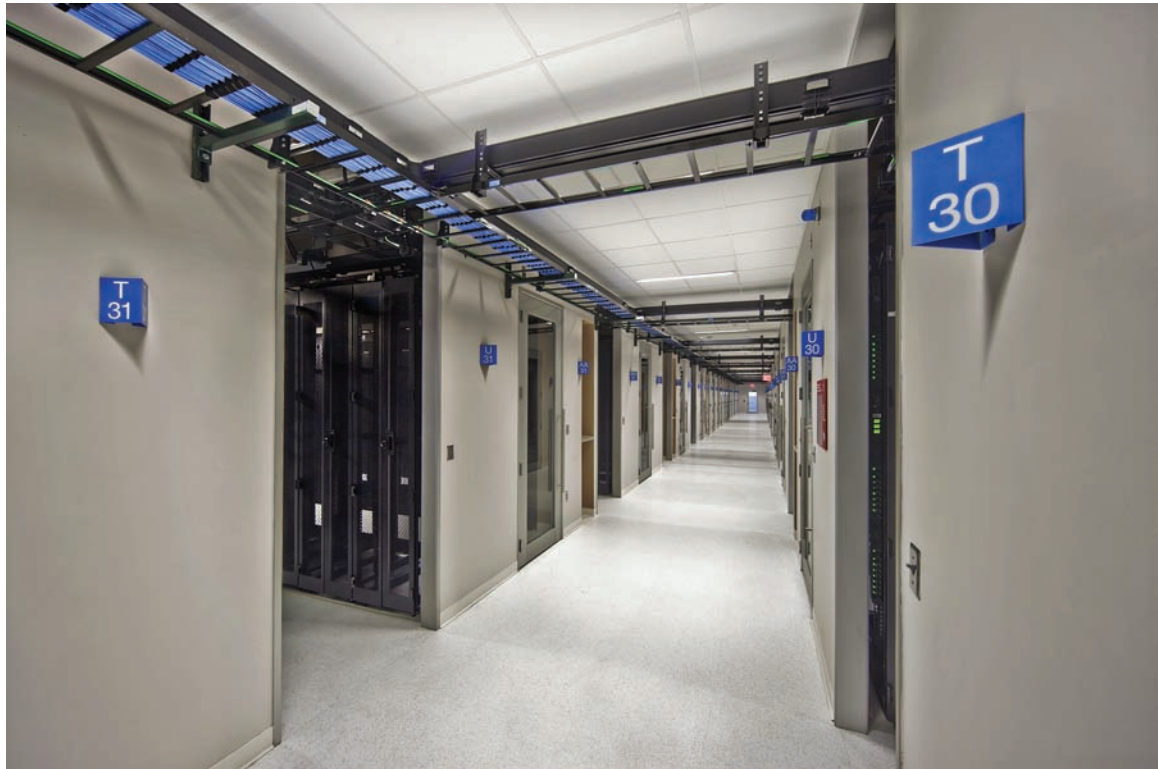
FIGURE 15-2 Cold room enclosures isolate hot and cold airflow for greater efficiency in NetApp's Research Triangle Park Data Center.
