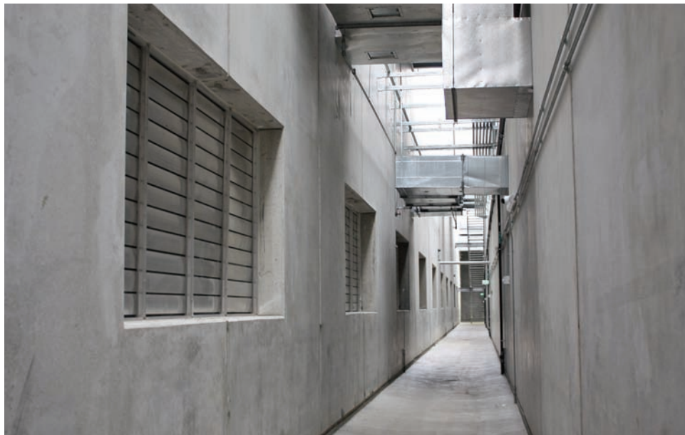
FIGURE 6-3 Adjustable louvers allow outside air to be brought into the Data Center. Image by Douglas Alger.
