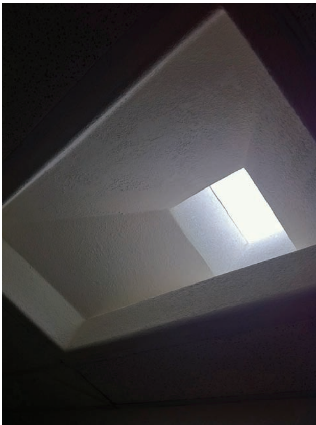
FIGURE 2-3 Solar tubing and skylights supplement the lighting in AISO's Data Center.
