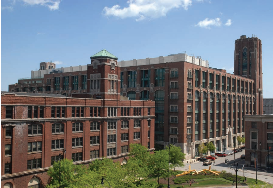
FIGURE 8-2 Built in the early 1900s as a printing plant, the building's strong floors and large vertical shafts made it an excellent candidate for conversion to hosting space.
