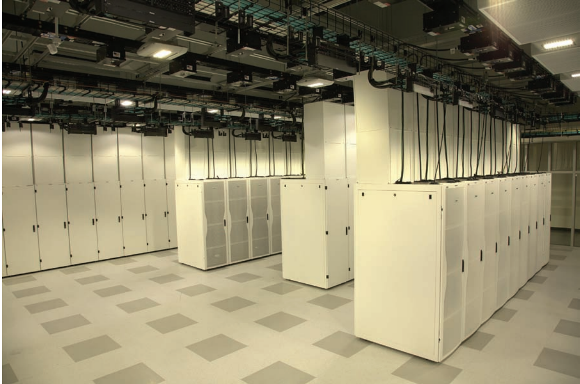
FIGURE 6-5 Enclosed cabinets with vertical exhaust ducts isolate hot and cold airflow, providing increased cooling efficiency. Image provided courtesy of Cisco. Photography by Cyclone Interactive.
