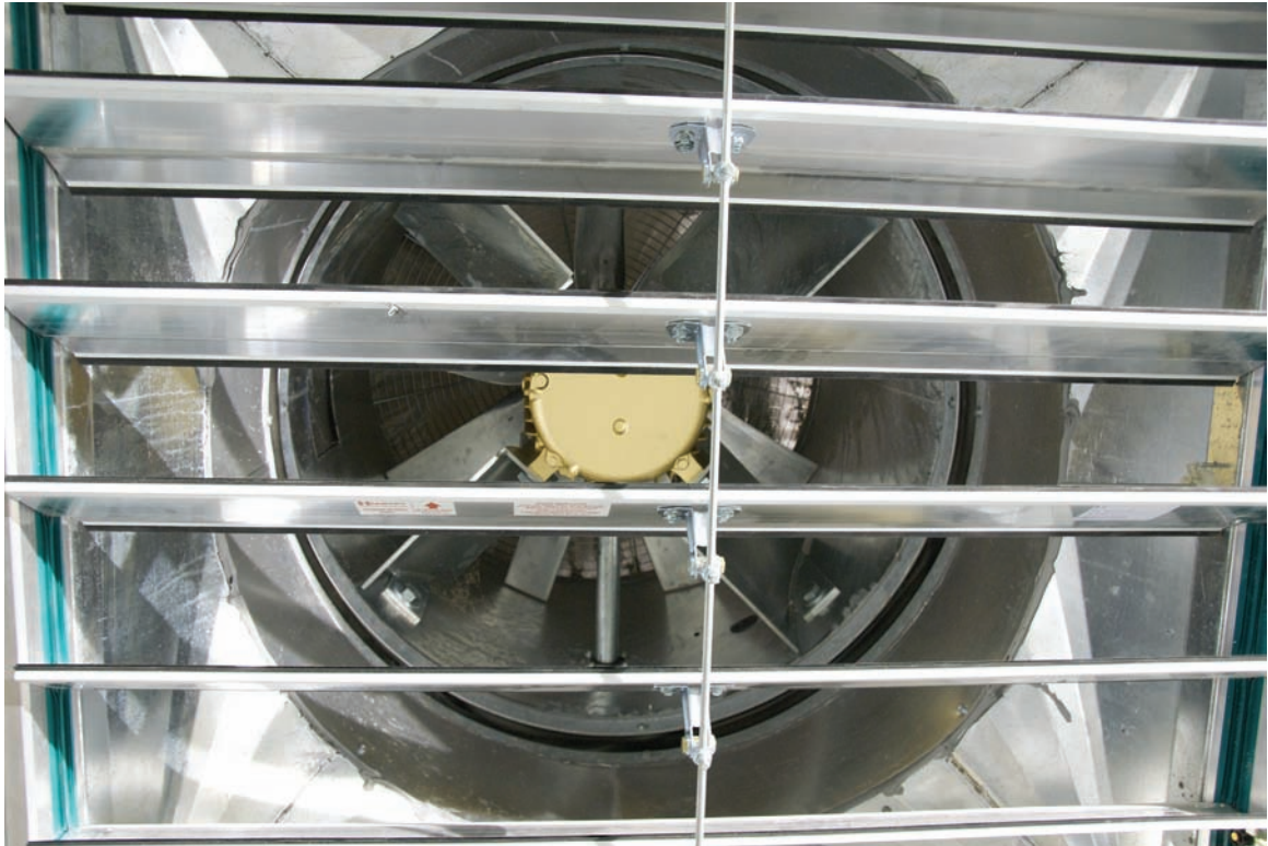
FIGURE 5-2 Variable drive blowers move air through Calcul Québec's Data Center at low velocity, consuming little power.
