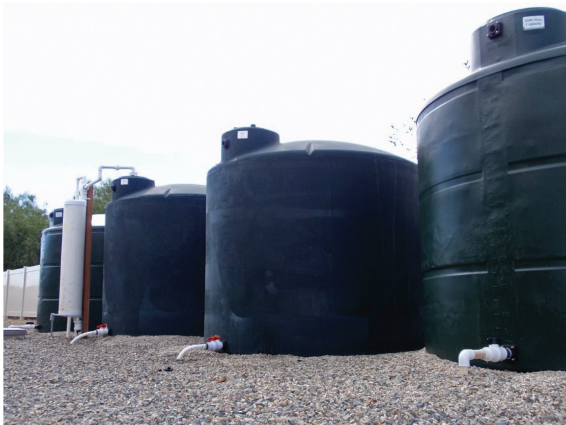
FIGURE 2-6 AISO harvests rainwater to cool its Data Center and for landscaping. Collection tanks can hold 10,000 gallons (37,851.1 liters) of water.
