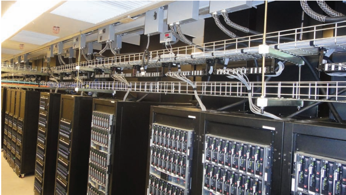
FIGURE 13-4 Structured cabling and electrical infrastructure are routed overhead in Intel's Data Center.
