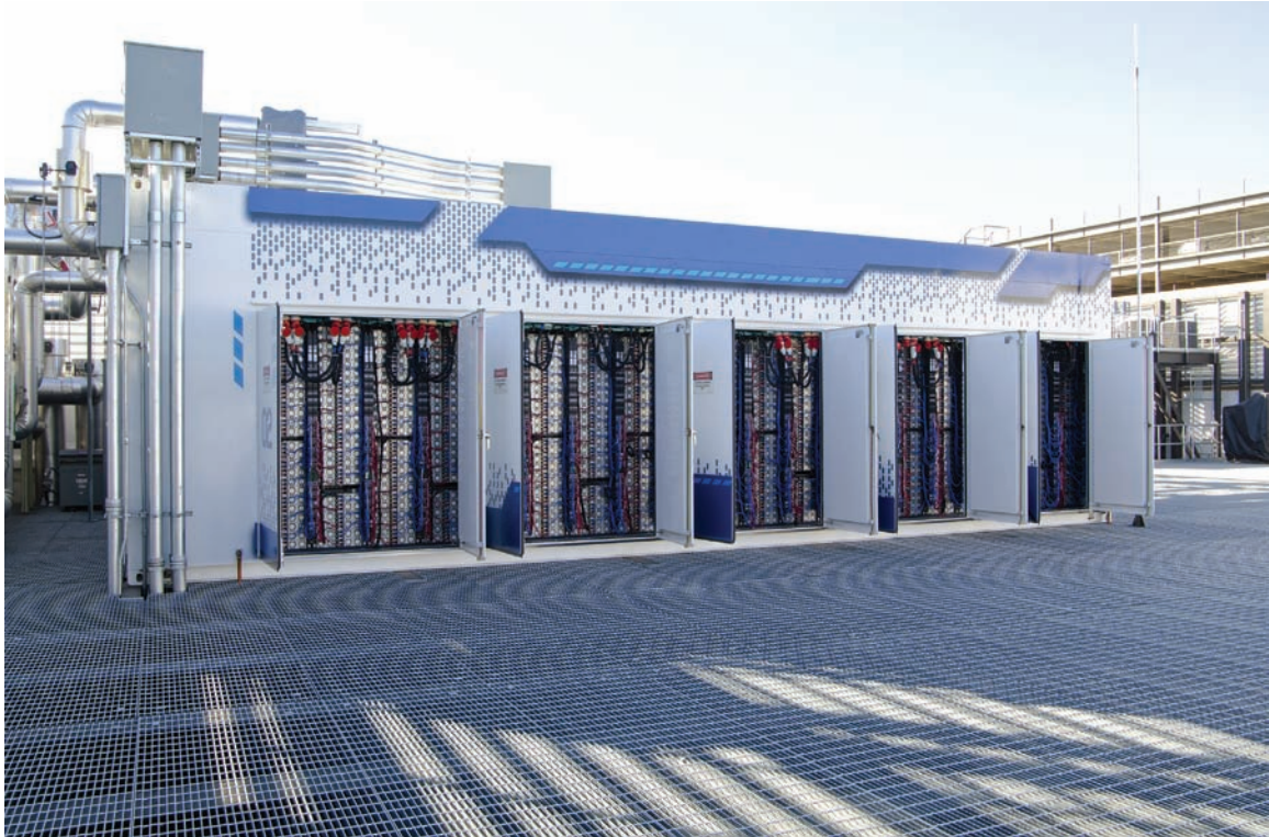
FIGURE 9-5 Half of the Data Center's capacity is provided by way of containers on the roof.
