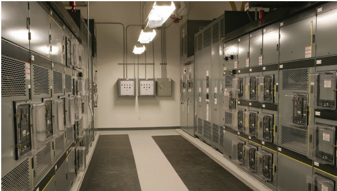
FIGURE 12-7 Electrical switchgear for IBM's Research Triangle Park Data Center.
