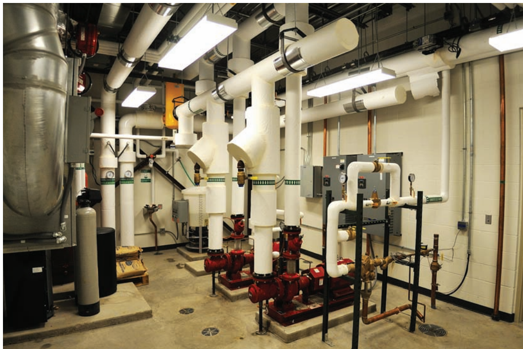
FIGURE 1-7 Chilled water piping for ACT's Iowa City Data Center. Image provided courtesy of KJWW Engineering Consultants.
