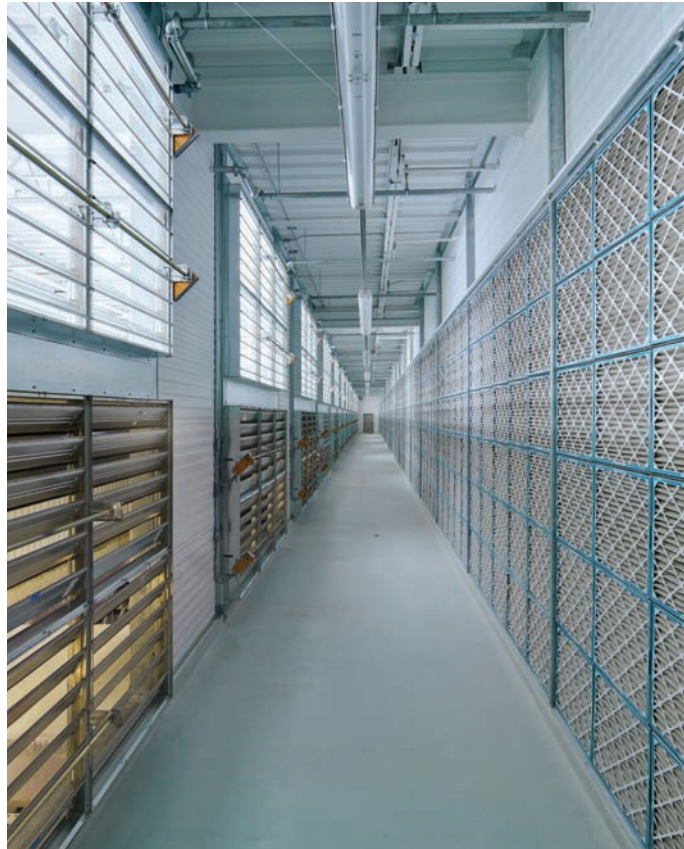
FIGURE 10-6 Outside air passes through multiple filters before entering Facebook's Data Center.
