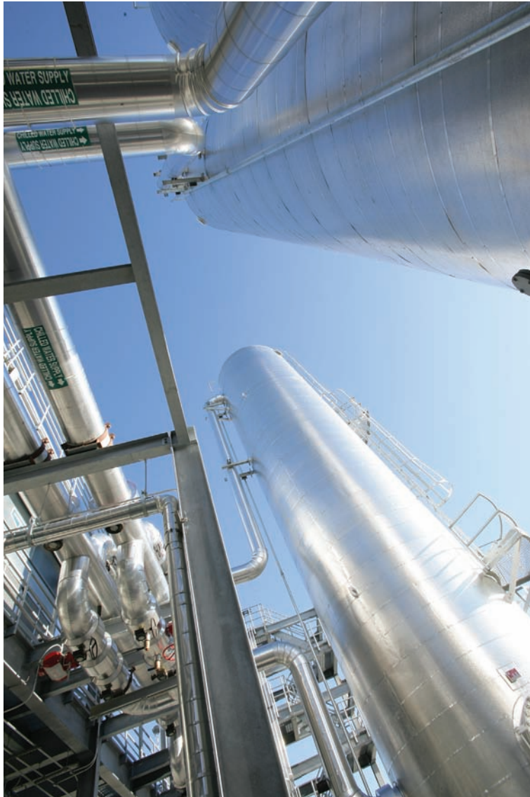
FIGURE 12-2 Thermal storage tanks for IBM's Research Triangle Park Data Center.
