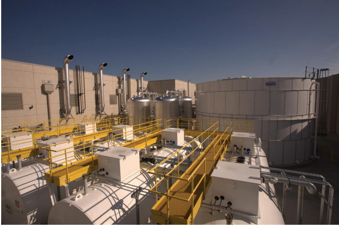
FIGURE 6-9 Four 20,000 gallon (75,708.2 liter) tanks of generator fuel, four 15,000 gallon (56,781.2 liter) tanks of chilled water, and one 355,000 gallon (1,343,821.2 liter) tank of domestic makeup water reside behind the Data Center. Image provided courtesy of Cisco. Photography by Cyclone Interactive.
