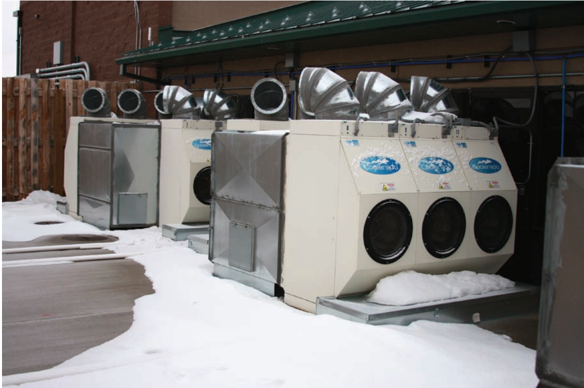
FIGURE 11-6 High-efficiency air conditioners cool Green House Data's Data Center.
