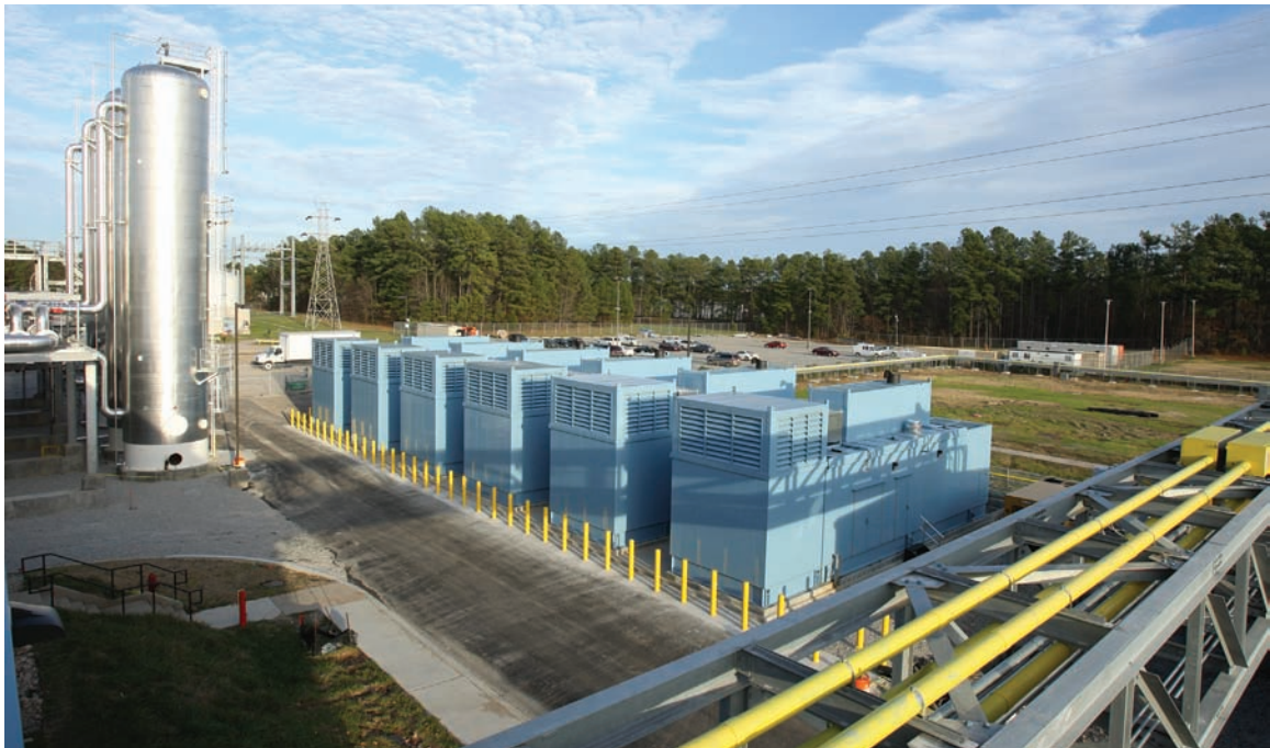
FIGURE 12-9 Six 2.5 MW generators provide standby power for IBM's Research Triangle Park Data Center.
