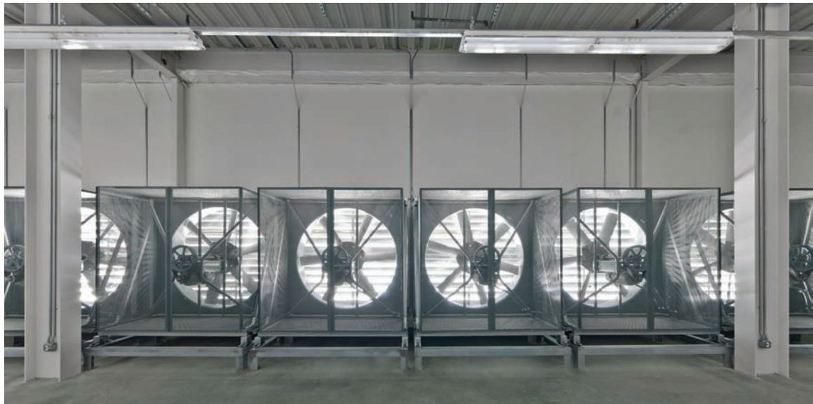
FIGURE 10-7 Mixing room fans.
