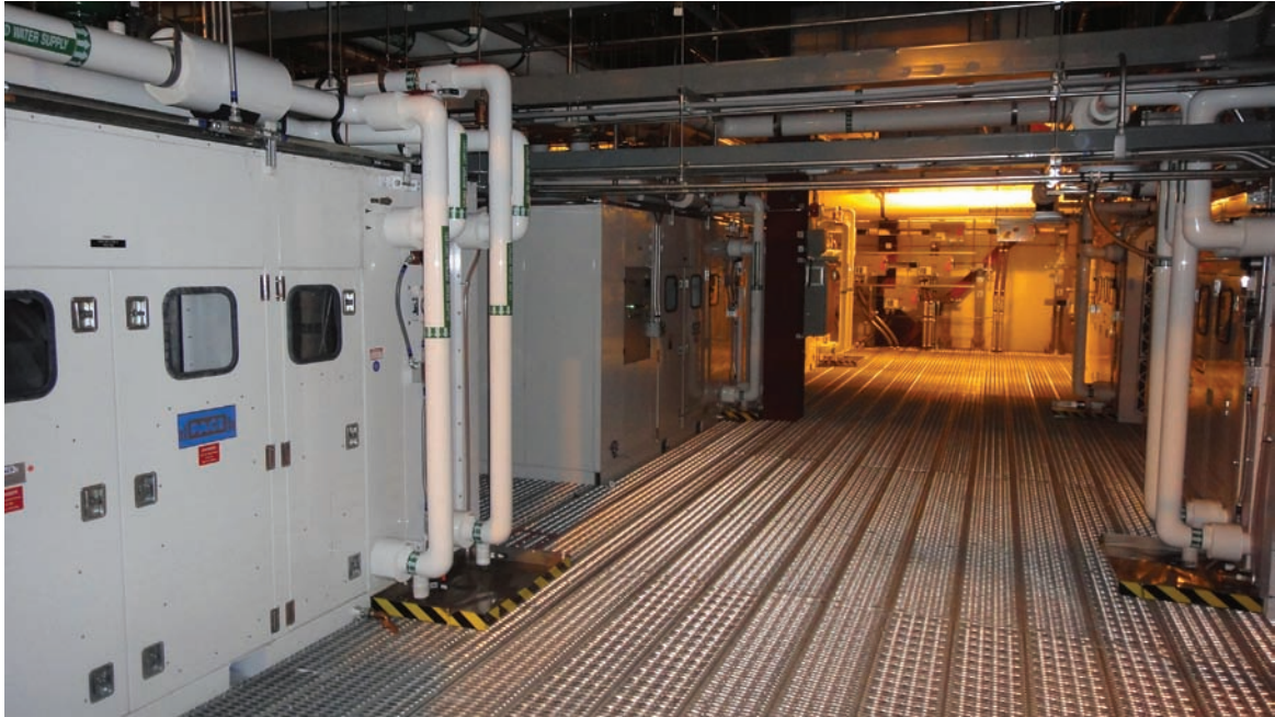
FIGURE 13-2 Air handlers on the third floor of Intel's Rio Rancho Data Center.
