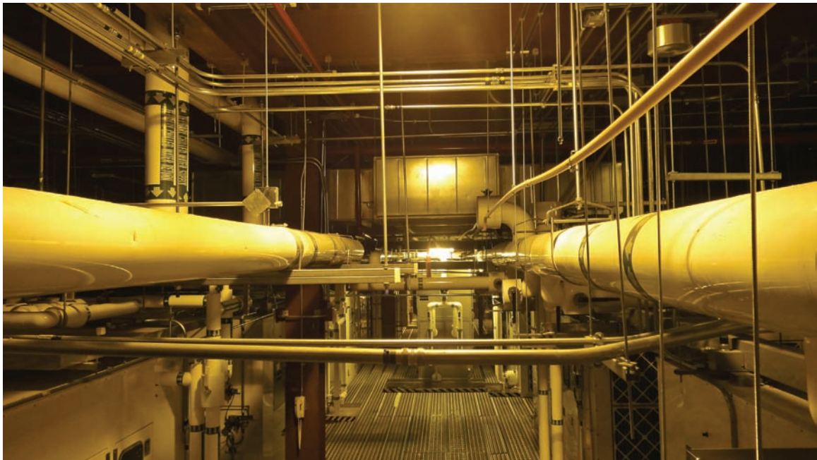
FIGURE 13-7 Chilled water piping.
