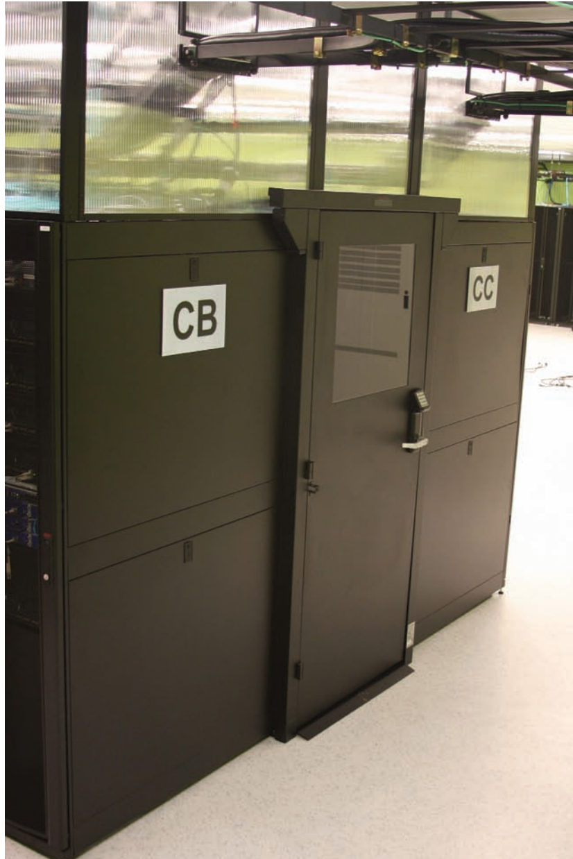
FIGURE 11-3 Plastic enclosures above the cabinets isolate hot and cold airflow while door panels control physical access.
