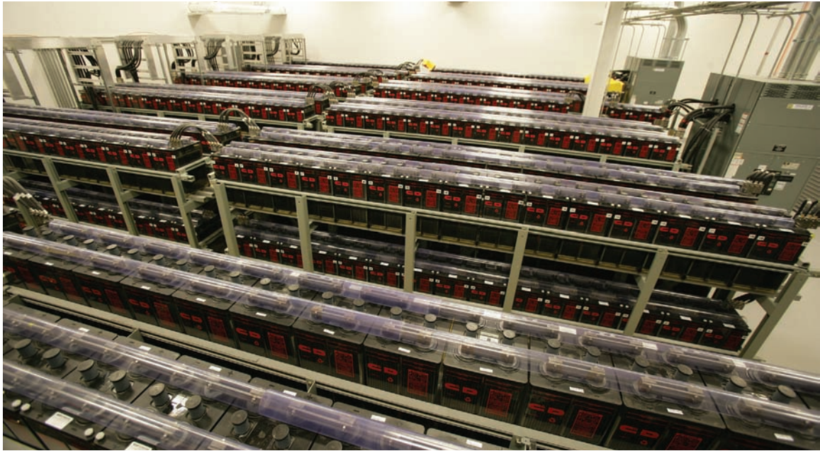
FIGURE 12-8 3 MW of wet cell battery capacity provide 15 minutes of ride-through power.
