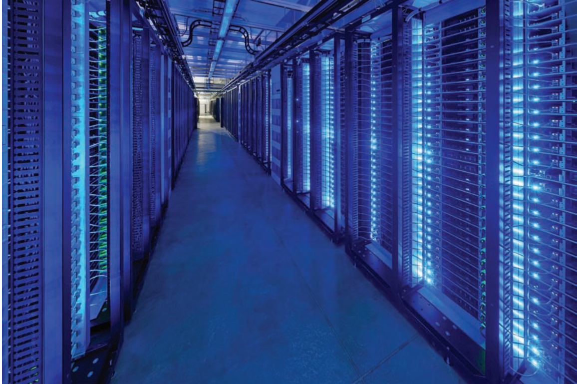
FIGURE 10-2 Facebook's custom servers feature no paint, logos, stickers, or front panel, eliminating weight and materials.
