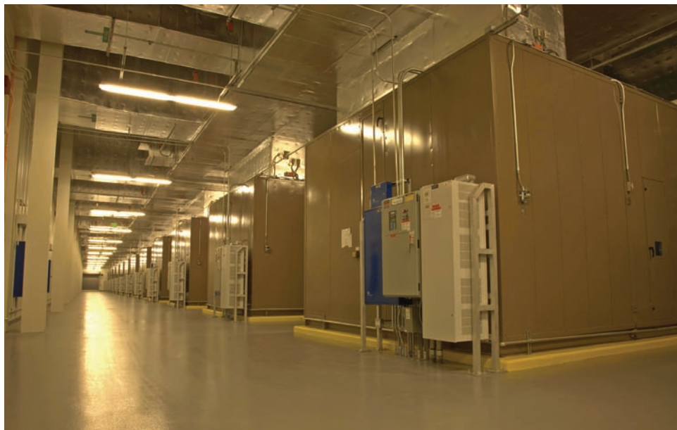
FIGURE 6-4 Thirteen air handlers feed cool air into a common plenum above the server rows. Airside economization allows the facility to be cooled by outside air more than half of the time. Image provided courtesy of Cisco. Photography by Cyclone Interactive.
