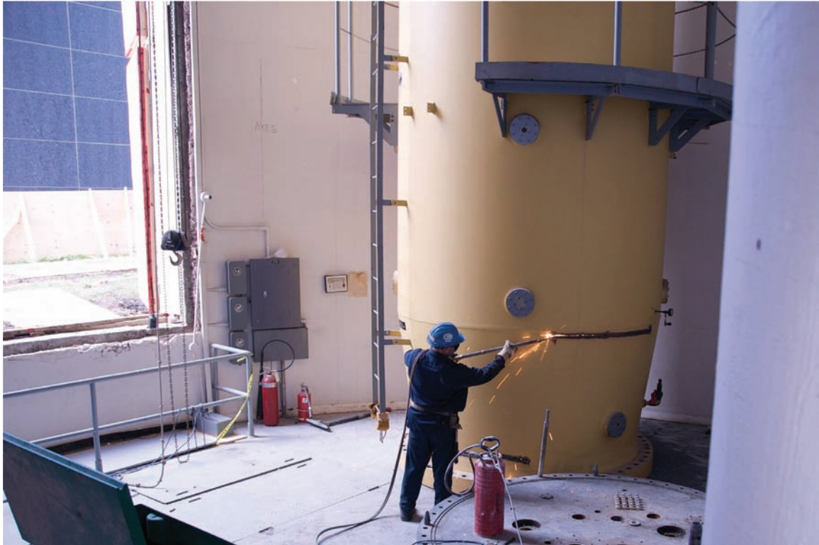
FIGURE 5-4 The housing for the Van de Graaff particle accelerator was sliced into rings to facilitate its removal. Shown here, the accelerator base rests on the floor.
