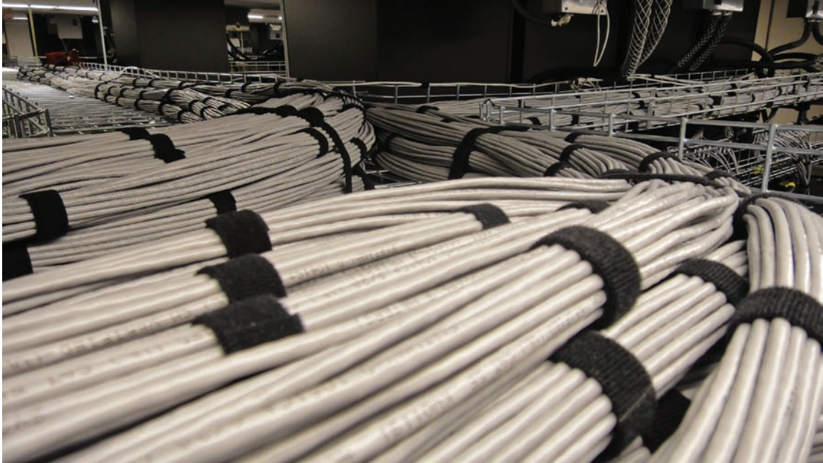
FIGURE 13-4 Structured cabling flows through an overhead cable tray in Intel's Rio Rancho Data Center.
