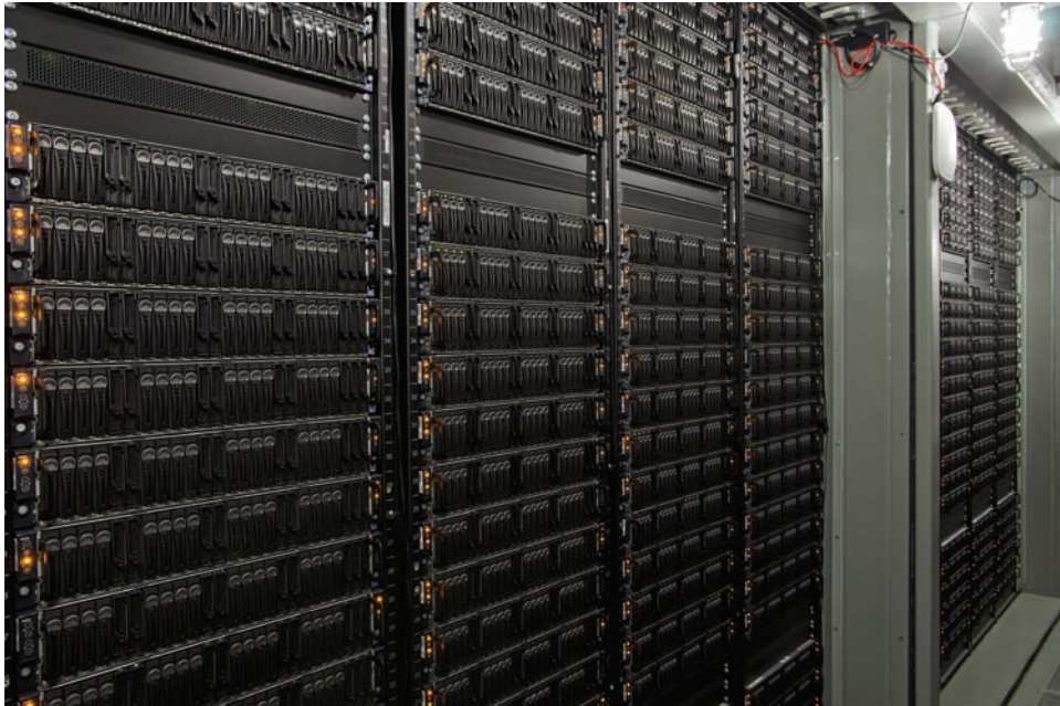
FIGURE 9-9 Containers are pre-populated with more than 1,500 servers each and then placed on the roof by a crane.
