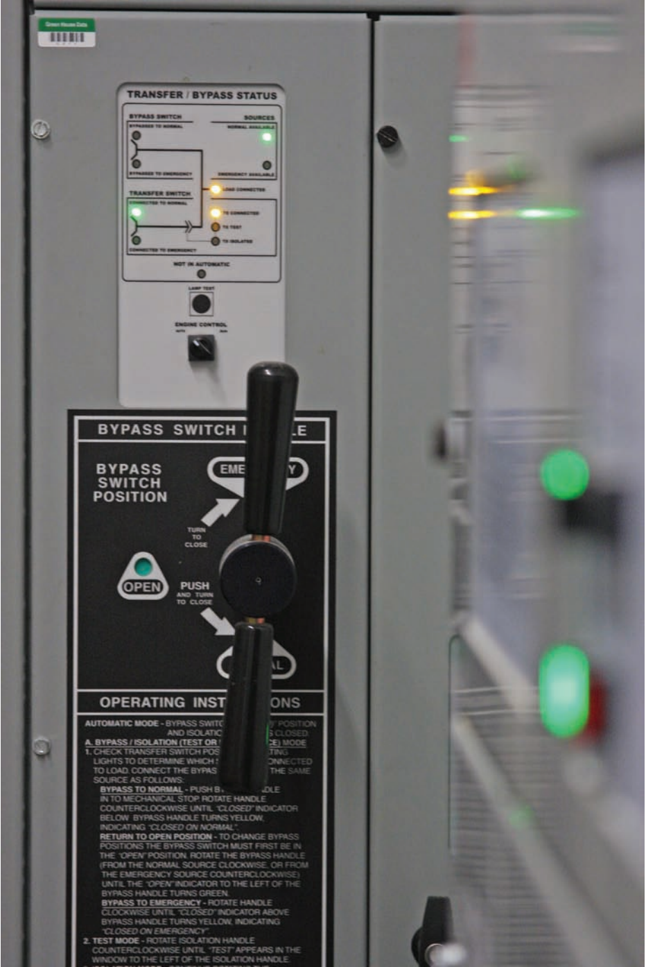
FIGURE 11-5 A closeup of the electrical bypass switch for Green House Data's server environment.
