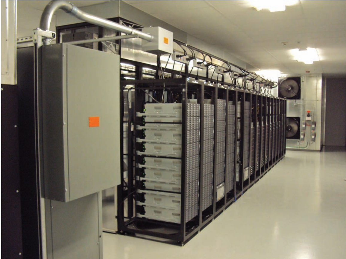
FIGURE 18-3 Power, cooling, and cabling infrastructure are delivered overhead to cabinet locations in Yahoo's Lockport Data Center.
