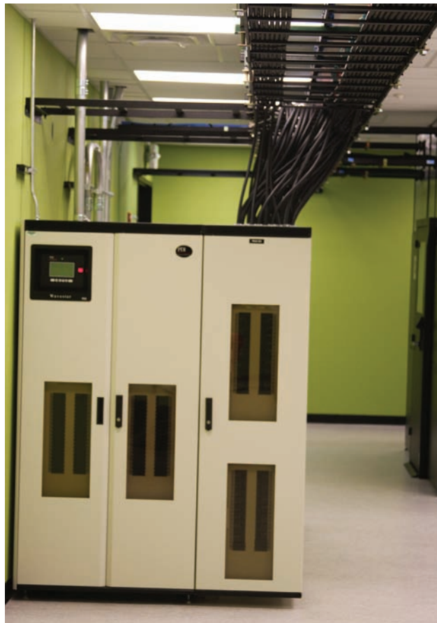
FIGURE 11-4 Power is distributed overhead to Green House Data's Data Center cabinet locations.
