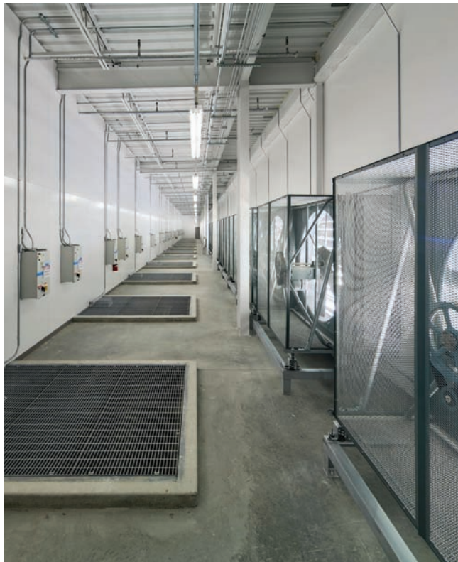
FIGURE 10-3 When needed, warm server exhaust is added to incoming air in a mixing room.
