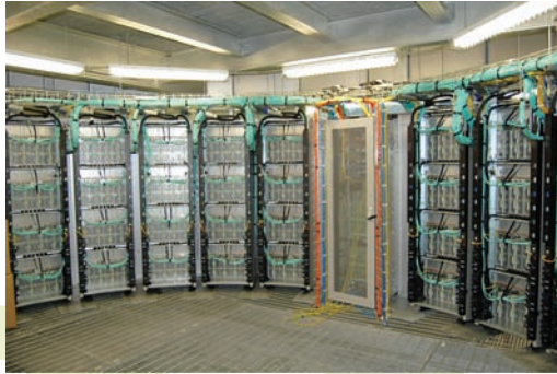
FIGURE 5-3 Hardware exhaust vents into a hot core and then is drawn down through the floor grating to cooling coils on the ground floor.
