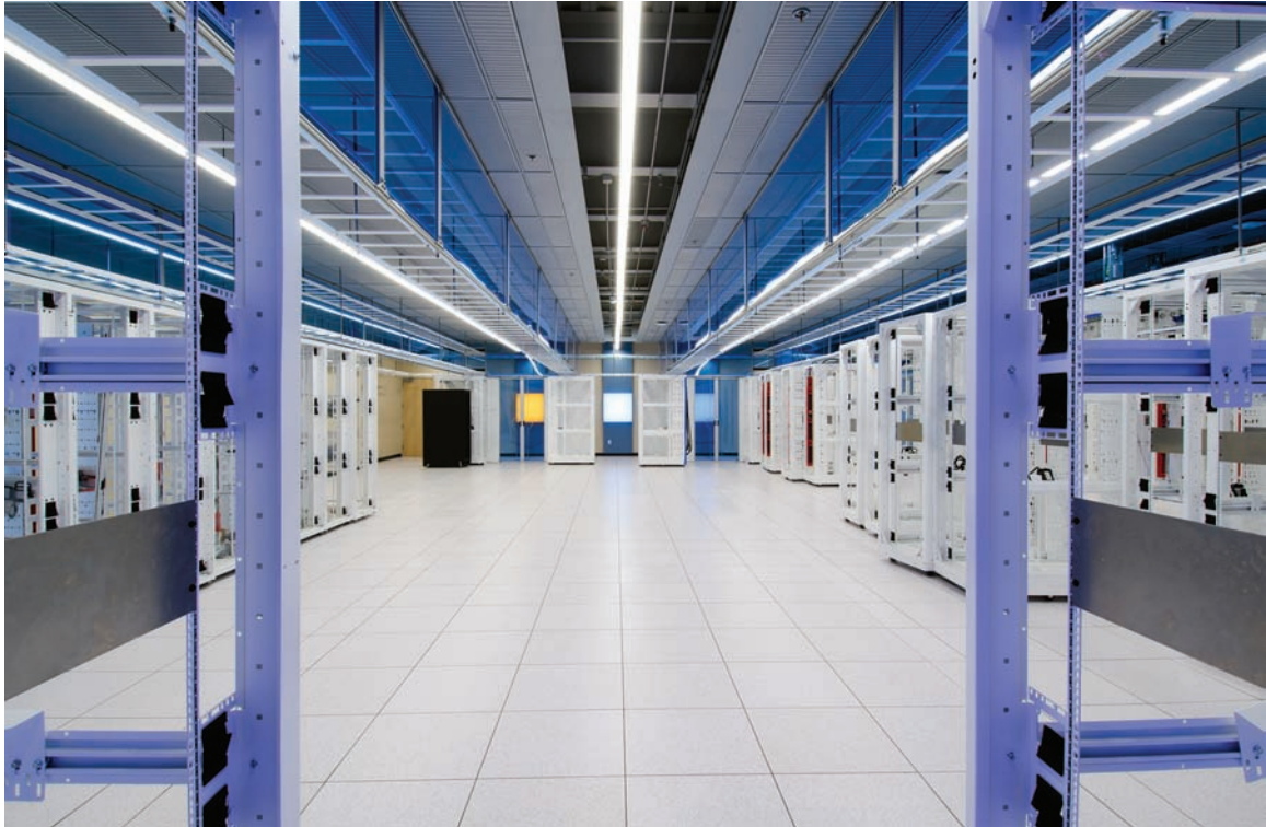
FIGURE 9-4 Liquid cooling piping is routed below a 6 ft. (1.8 m.) raised floor while power, cooling, and cabling are distributed overhead in eBay's Project Mercury Data Center.
