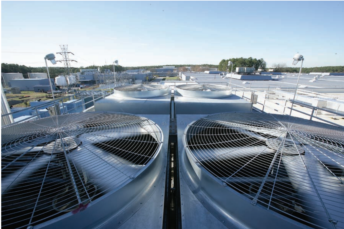
FIGURE 12-10 Cooling tower fans for IBM's Research Triangle Park Data Center.
