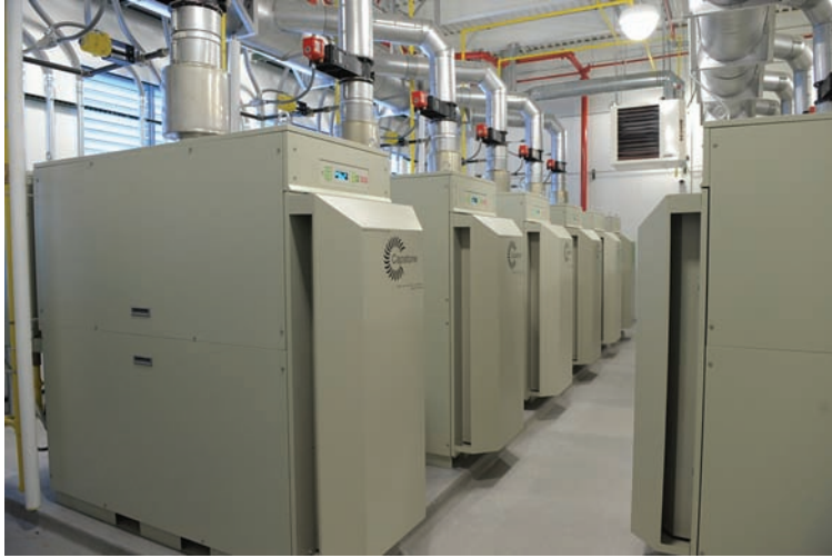
FIGURE 16-3 Primary power for Syracuse University's Data Center comes from twelve 65 kW hybrid UPS microturbines.
