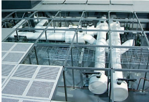
FIGURE 12-3 Pre-piping under IBM's raised floor supports future water cooling in the Data Center.
