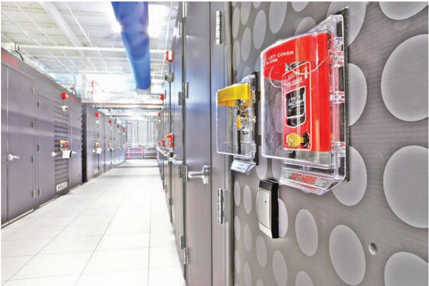
FIGURE 14-10 Fire suppression controls and a badge reader adorn the side of a Data Center module.
