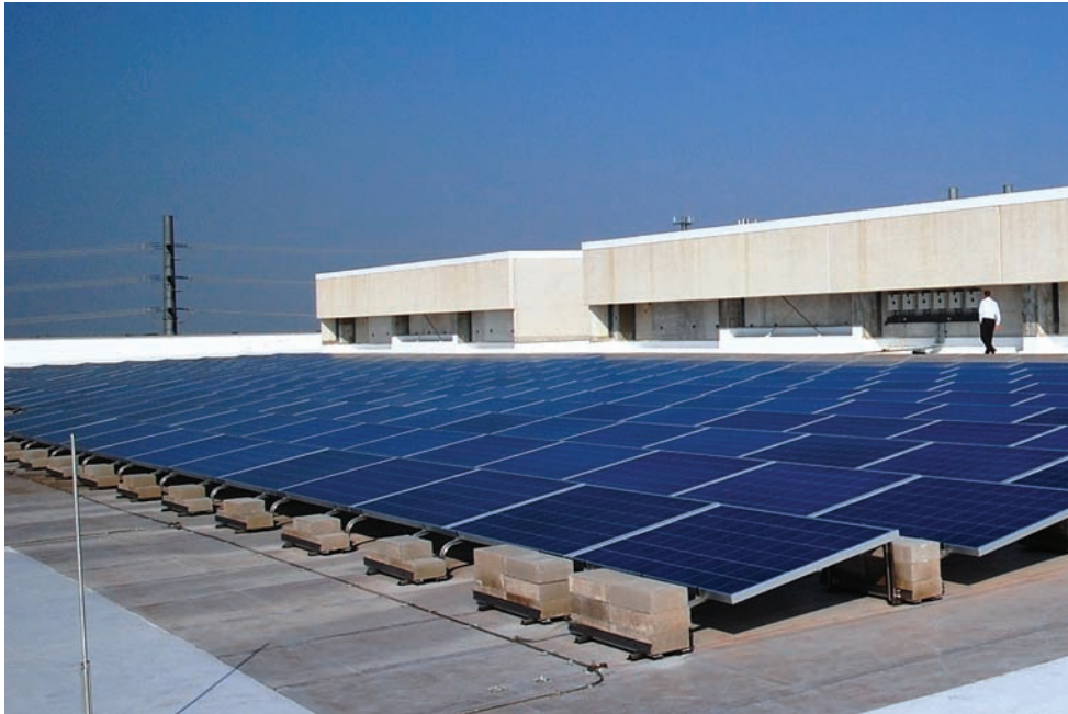
FIGURE 6-7 A 100 kW rooftop solar panel array provides enough energy to power the office area for personnel who support the Data Center. Image by Andrew Broer.
