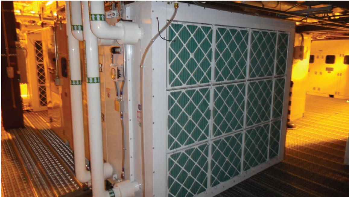
FIGURE 13-6 One of the air handlers supporting the Rio Rancho Data Center.
