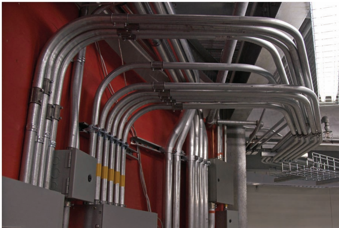
FIGURE 5-8 Power and cabling infrastructure are delivered overhead to cabinet locations on three floors.
